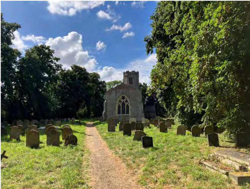
Plate 23: View of St Catherine's Church, Fritton within Fritton Conservation Area, facing west
