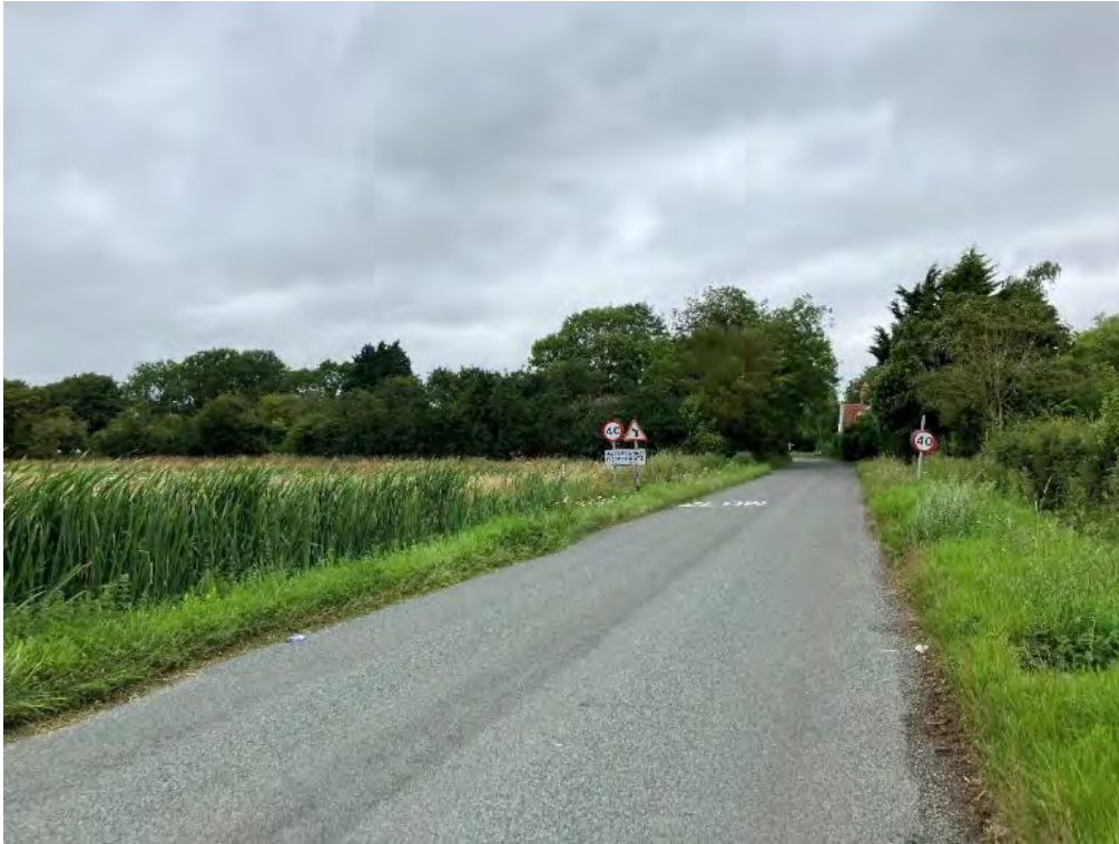
Plate 41: View from Sub-Site 7D looking towards the eastern end of Saxlingham Green Conservation Area, Manor Farmhouse and Manor Cottage (both not visible) and Manor Farmhouse Barn, facing north
