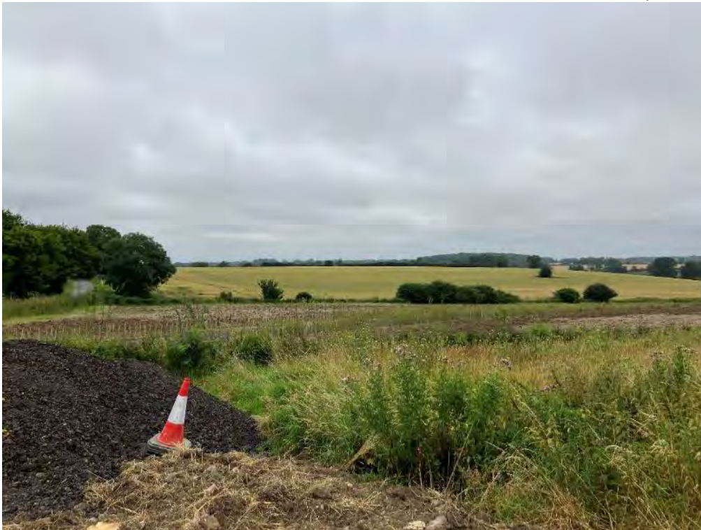
Plate 49: View from Upgate Green Farmhouse and Outhouse looking towards Sub-Site 8B, facing south
